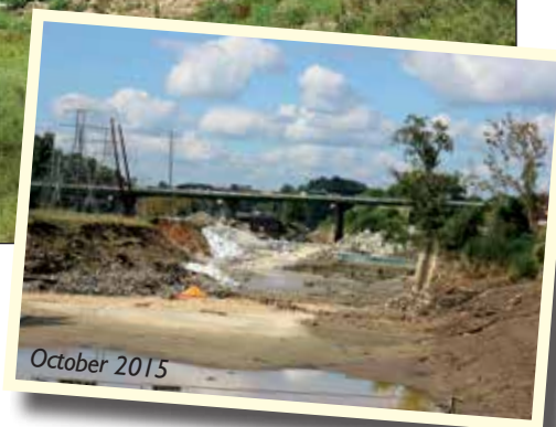
Temporary repairs to the breached Columbia Canal dike remain visible in September 2016.
