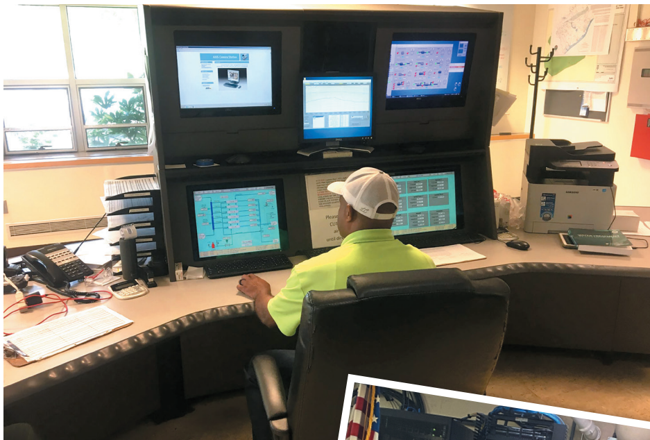
Above: Jermaine Holmes, water operator for the City of Florence, monitors groundwater pumps, elevated tank levels and surface water treatment filters in the control room at the city’s Surface Water Treatment Plant. Photo: City of Florence.
