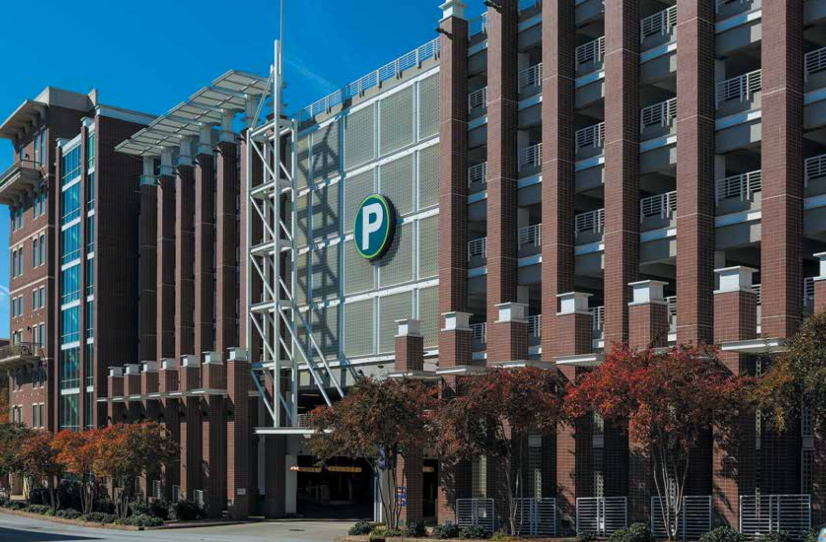
South Spring Street Garage, Greenville
