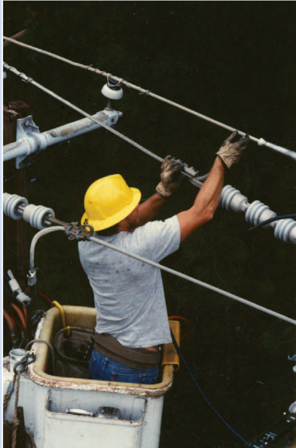
As part of the South Carolina Association of Municipal Power Systems mutual aid program, linemen from municipal electric utilities in South Carolina and neighboring states work to restore power in Camden, Orangeburg, Rock Hill and Georgetown, all municipal power cities.
