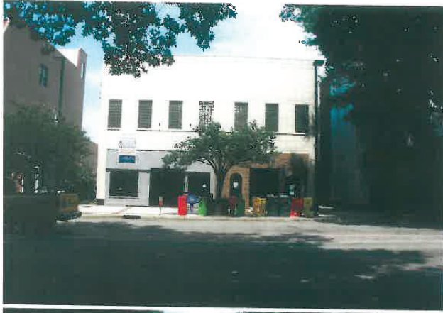
← 1520 & 1522 MAIN - BUILDING TO BE DEMOLISHED - SITE OF PROPOSED PROJECT
