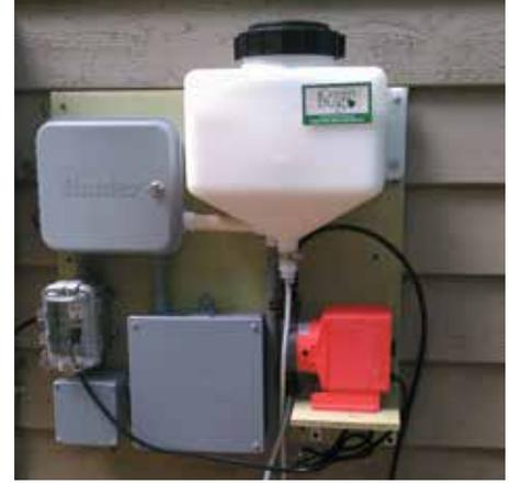
*The Greenbug Injector System uses an existing irrigation system to distribute Greenbug for Outdoors so that anywhere water is directed becomes safely pest free.*
