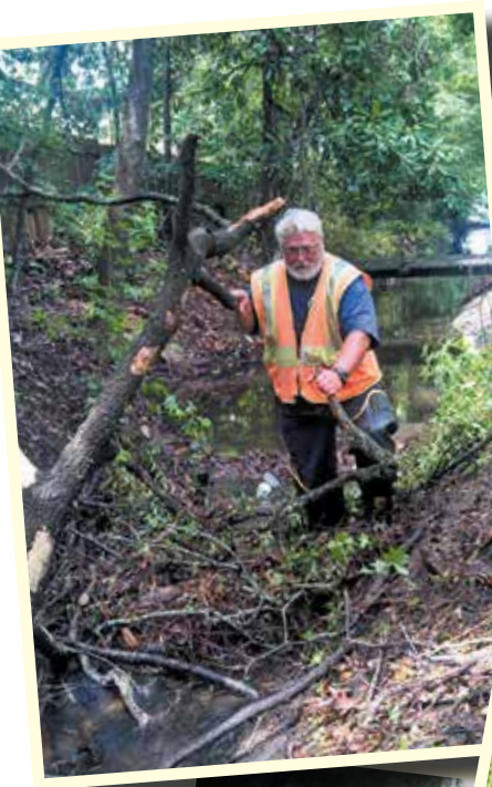
Continuous attention to clearing drains and pipes is part of Mount Pleasant's recipe for success.
