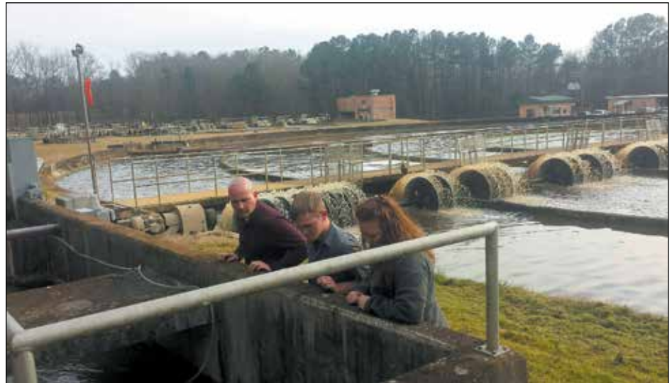
Town Manager Ted Luckadoo and Batesburg-Leesville utility staff inspect the town’s new liquid lime chemical feed system.
