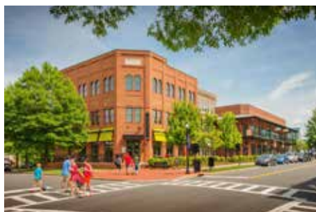
Form-based codes emphasize building frontages, creating places like Baxter Village in Fort Mill.
