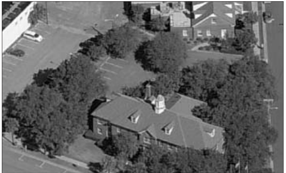
A pictometry image of Myrtle Beach City Hall taken in May shows three-dimensional detail of the building and surrounding structures.
