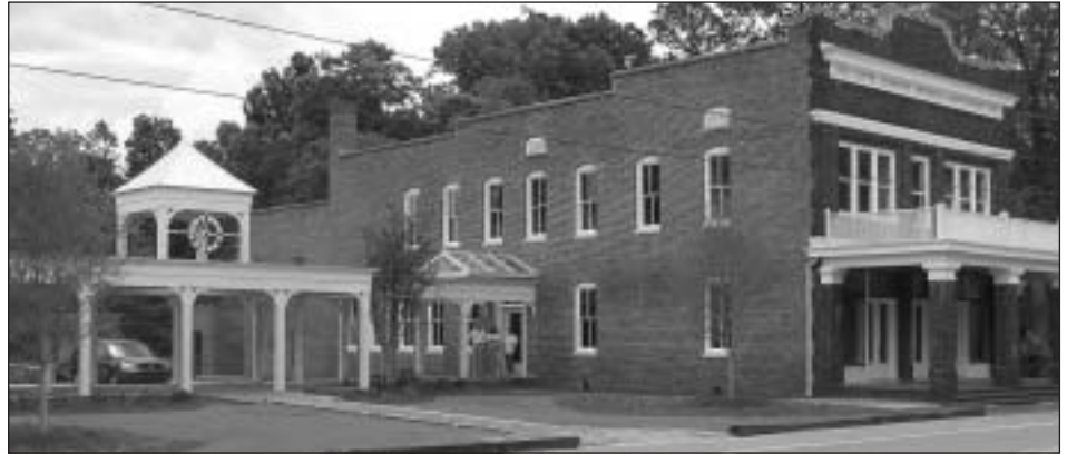
The initial phase of "Meggett 1925" was the construction of the Donor's Pavilion that connects town hall and an adjacent Town-owned building.
