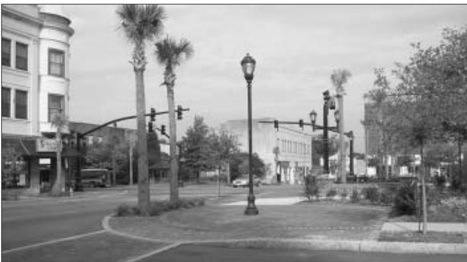
Once complete, the City of Orangeburg’s Streetscape Project added underground utilities, trees and plantings, and period street lighting.
