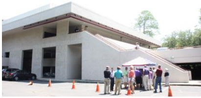
Example of bad lighting
